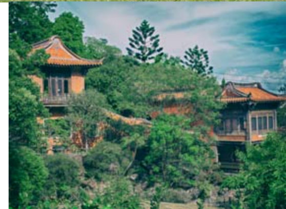
Buildings in the traditional southern Chinese Jiangnan style overlook a landscaped garden in the Nanyuan Land of Retreat and Wellness resort in Hsinchu County. PHOTO: PAUL COOPER, TAIPEI TIMES
